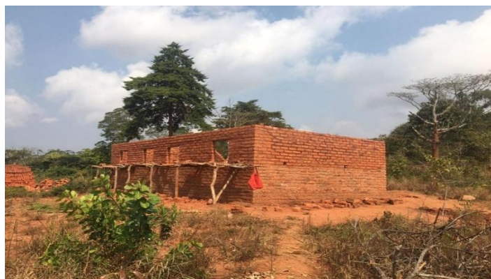
Figure 1. The construction in progress of Chisomo ECD in progress, captured September 2025
